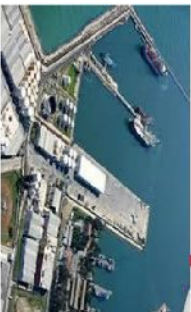
BP ATAŞ Dolum Tesisi BP ATAŞ Loading Facility
