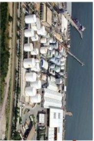
Socar Rafinerisi Socar Refinery
